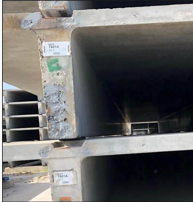
InfoSight Tag applied to precast concrete products
