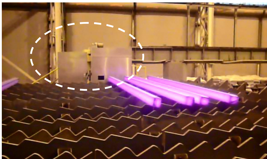
Tag Nailer installed at fixed station of cooling bed (Note - color of bars is due to radiant infrared color shift)
