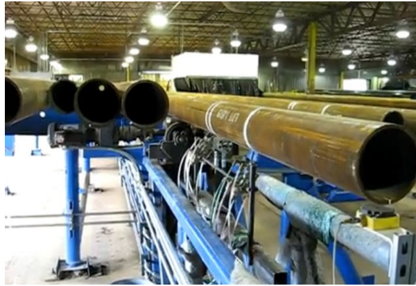
Example of under-the pipe nozzle mounting at spin roll station
